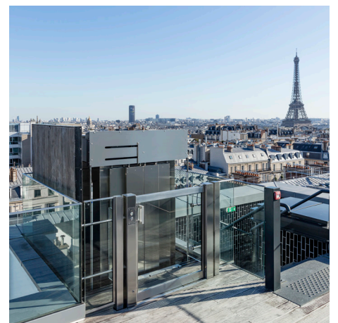
The flap has opened, the lift cabin rises.
