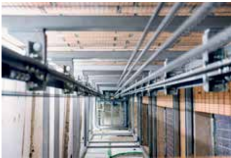
The fitted steel frame extends through all floors.
